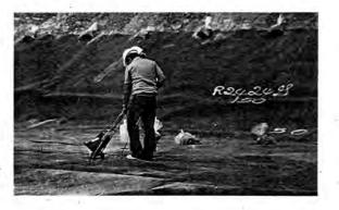
The Westinghouse landfill will include two synthetic liners similar to the one being installed here. The synthetic liners are an integral part of the landfill's advanced collection and monitoring system that will virtually eliminate the potential for leaks.
