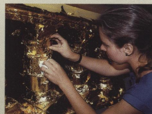
RESTORING GILDING ON BALUSTERS, 1988
